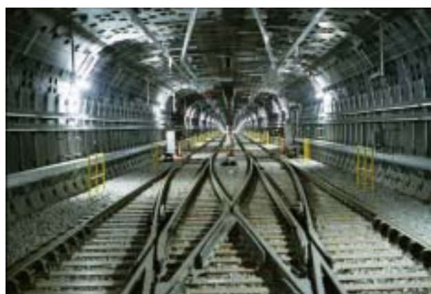
Photo 5: Completed crossover section (March, 2004)
