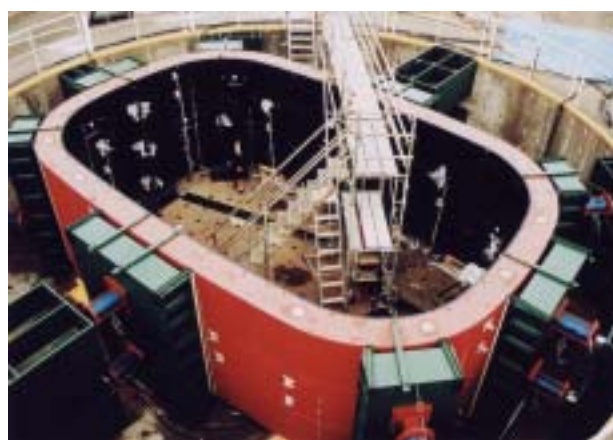
Photo 1: Assembled-segments test on composite segment rings
