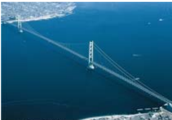
Photo 3: Akashi Kaikyo Bridge
