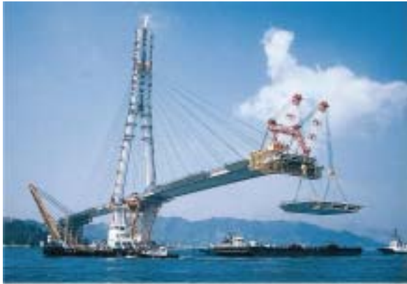
Photo 11: Overhang construction of the girder (Tatara Bridge)
