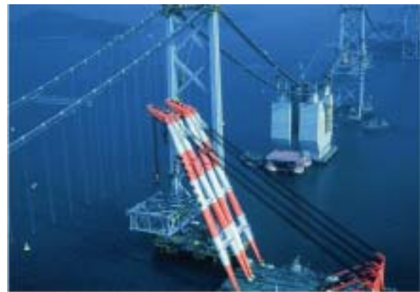
Photo 8: Large block construction for the stiffening girders (Seto Ohashi Bridge)
