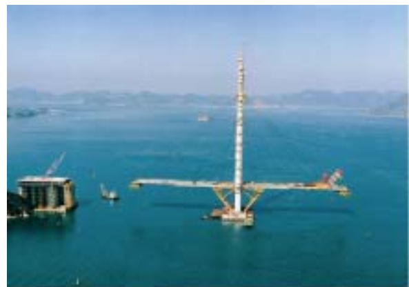
Photo 10: Balancing construction of the girder (Tatara Bridge)
