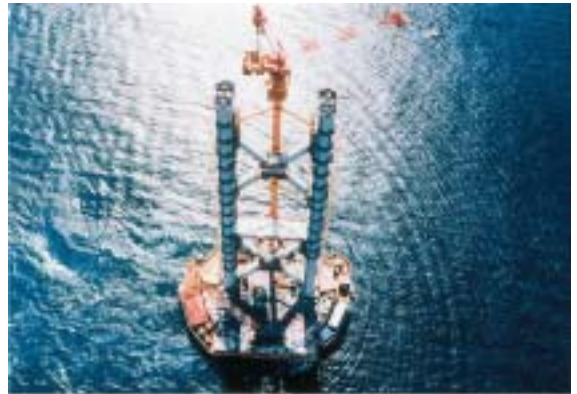
Photo 6: Tower construction using a tower crane (Akashi Kaikyo Bridge)
