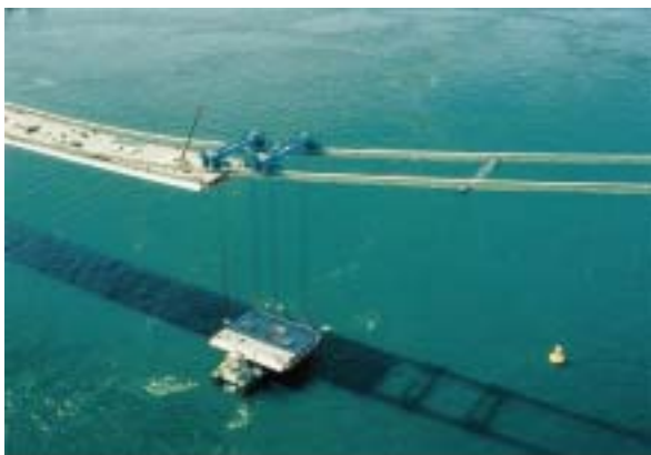
Photo 9: Girder construction using a self-positioning barge (Kurushima Kaikyo Bridge)
