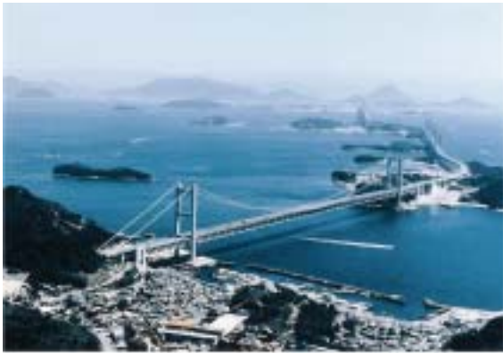
Photo 2: Seto Ohashi Bridge
