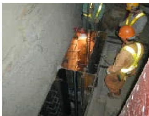
Photo 2: Constructing JES toward Length
