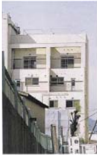
Photo 4: Restored apartment building
