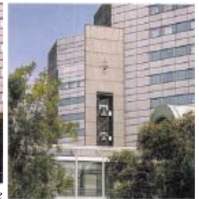
Photo 6: Restored clock tower
