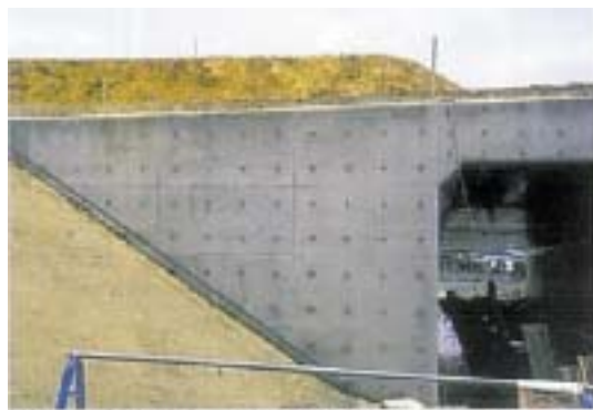
Photo 2: Box culvert after the repair
