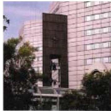
Photo 5: Clock tower tilted due to an earthquake
